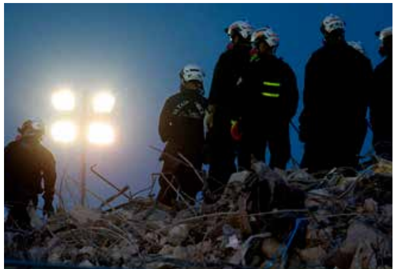
Working the pile.
