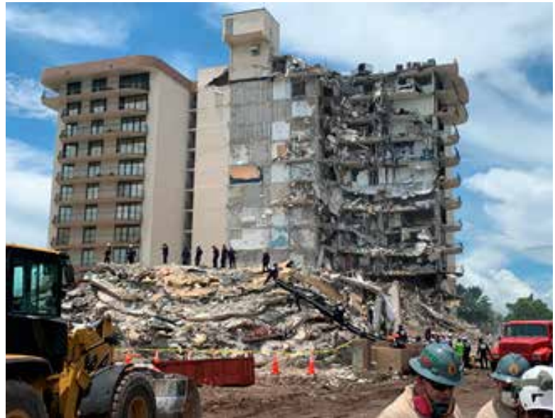
The site of the Champlain Towers South partial collapse in Surfside, Florida. Credit: NIST
